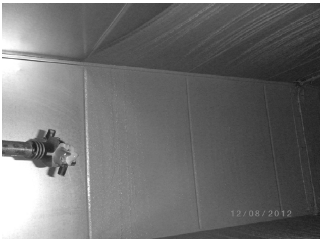
Figure 14: Class A robotic application of sealant.
