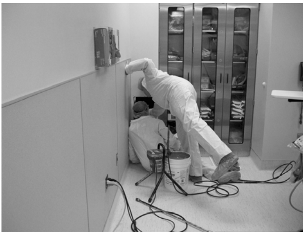
Figure 13: Manual sealing around a service opening.
